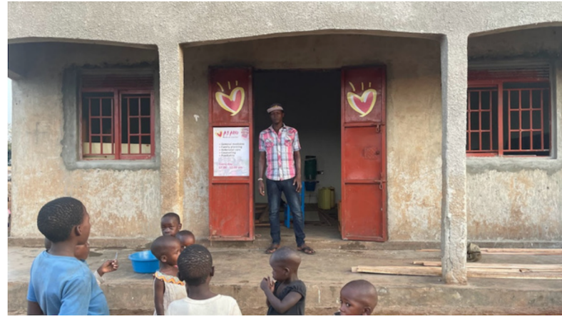
The building yet to be painted.
