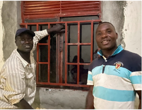
The builders installing windows
