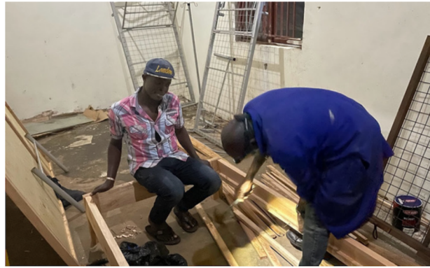
The carpenter partitioning the medical center
